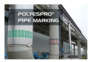
PolyesPro<sup>®</sup> Pipe Marking film is a high performance non-PVC polyester sandwich, manufactured according to 3M<sup>™</sup> MCS<sup>™</sup> (Matched Component System<sup>™</sup>) production specifications.
