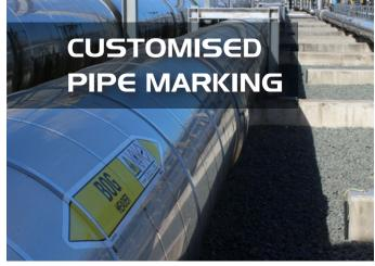
Within our production process we can make several different layouts of pipe marking. These layouts always include the mandatory (in most national norms & regulations) safety information:
